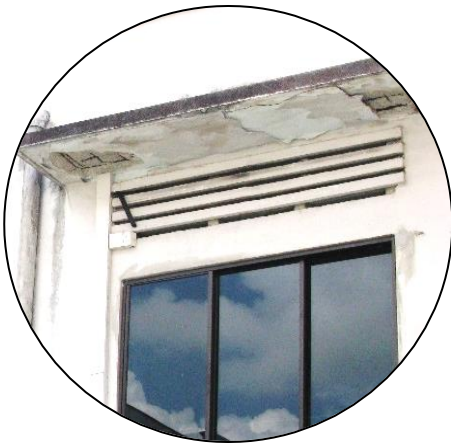
Spalling concrete
