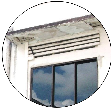
Spalling concrete
