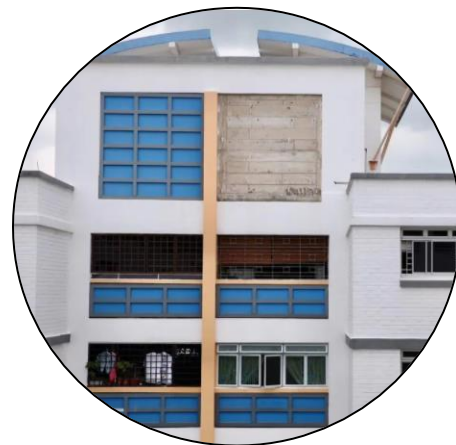
Dislodged metal cladding
