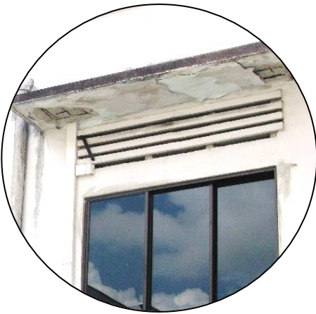
Spalling concrete
