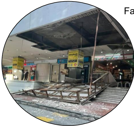
Collapsed exterior ceiling
