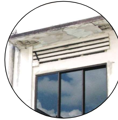
Spalling concrete
