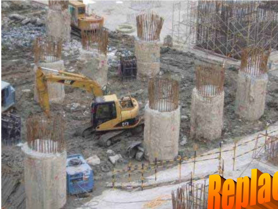
Bored cast-in place piles
