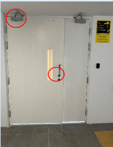
Figure H—VII: One-way lock and self closing door / gate; with a signage to indicate maintenance area
