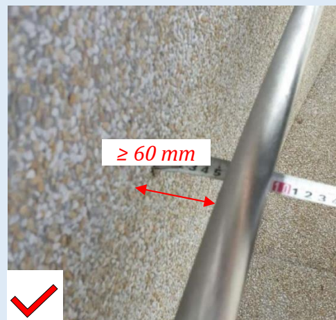
Figure E—XVIII: Clear space from rough wall surface (Min. 60mm wall gap)
