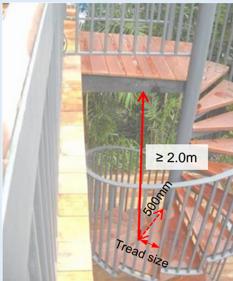
Figure E—IV: Measurement of headroom for a spiral staircase
