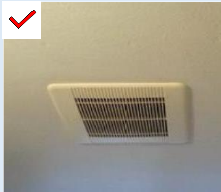
Figure G—IV: Ducted fresh air supply outlets
