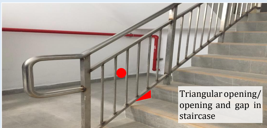
Figure H—XXVI: Opening or gap size in a flight of staircase
