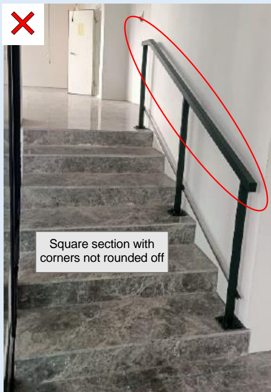
Figure E—XV: (Photograph 1) Unacceptable handrail profile
