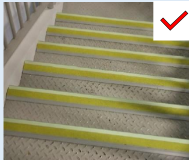
Figure E—XXV: Nosing provision for perforated metal staircases at maintenance areas
