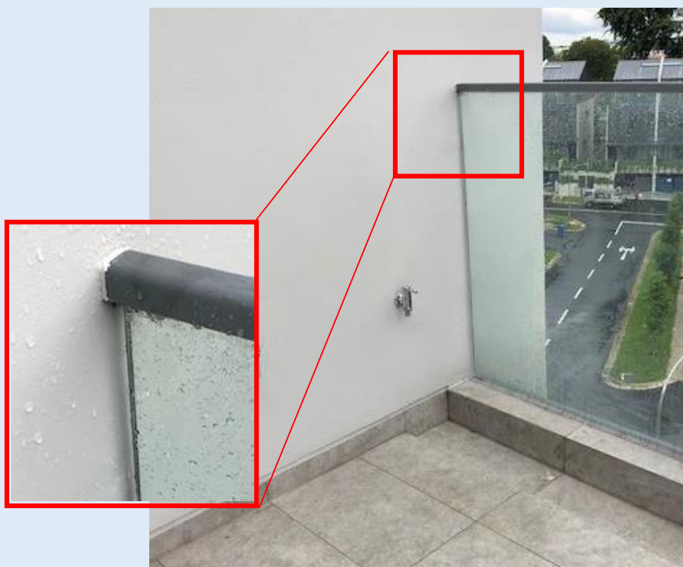
Figure H—XXXV: An example of glass barrier with continuous rail fix to top edge of glass
