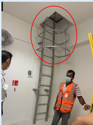
Figure H—VIII: Locked-entry cat ladder / hatch doors; with signage to indicate maintenance area
