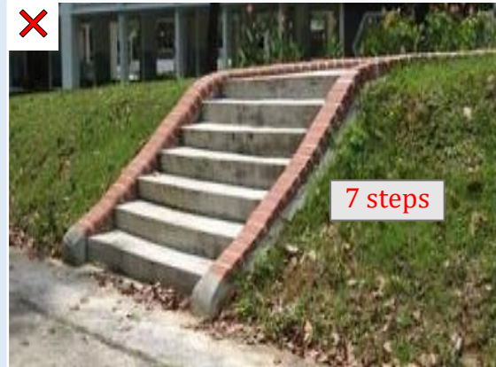
Figure E—XI: Photos from site inspections that depict staircase which are not provided with handrail
