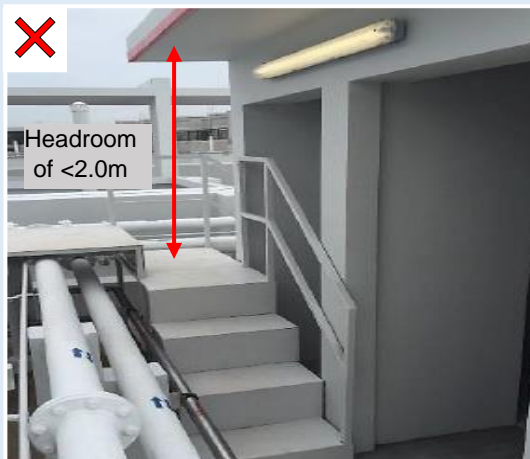
Figure C—V: Steel staircase was rectified to increase headroom space
