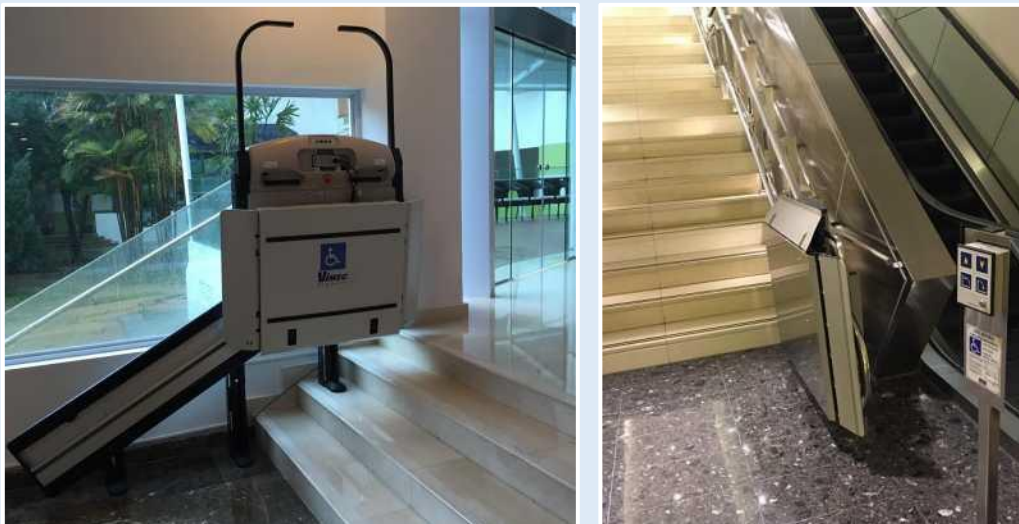
Figure K—II: Examples of stairlifts
