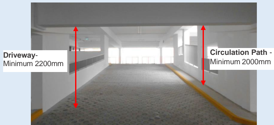
Figure C—IX: Comparison of headroom measurements on the driveway and circulation path
