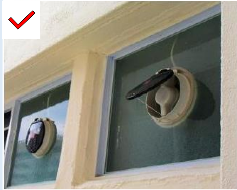
Figure G—III: Window or wall mounted fan
