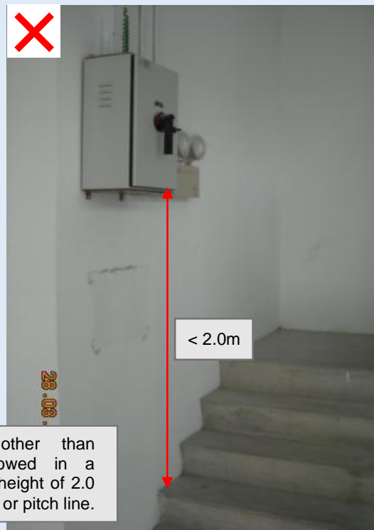
Figure C—XVII: Examples of headroom non-compliances along staircases
