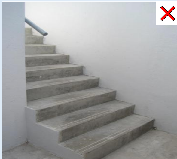
Figure E—XX: Non-continuous handrail
