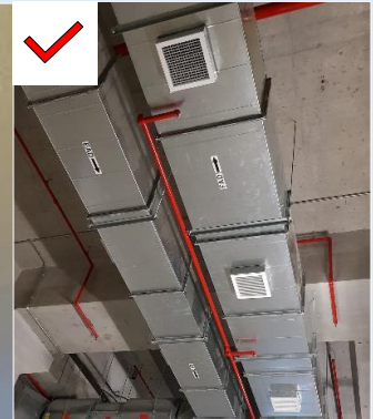
Figure G—IV: Ducted fresh air supply outlets
