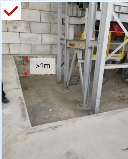
Figure H—XII: M&E floor openings without barriers
