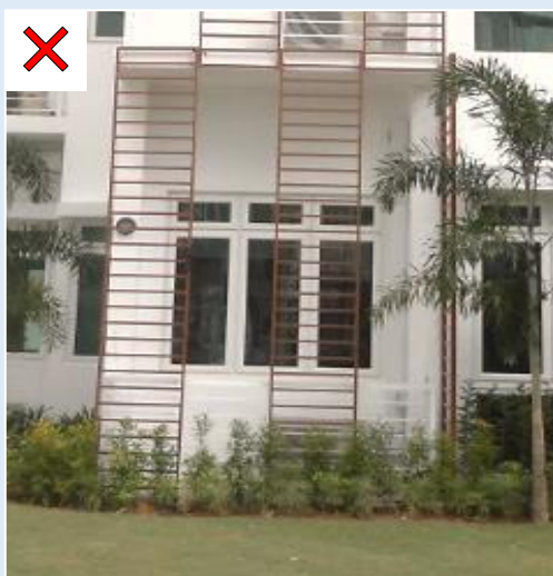
Figure H—I: Climbable features posing risk of falling from height
