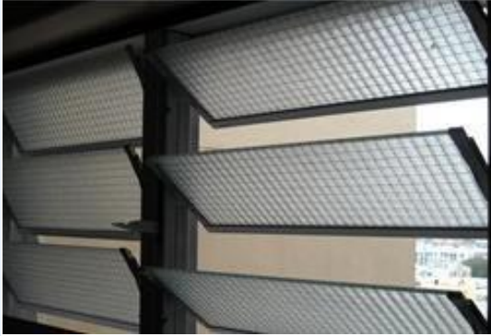
Figure G—IX: Openings in adjustable louvres
