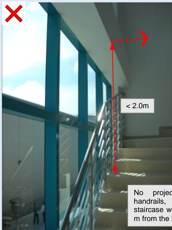
Figure C—XVII: Examples of headroom non-compliances along staircases
