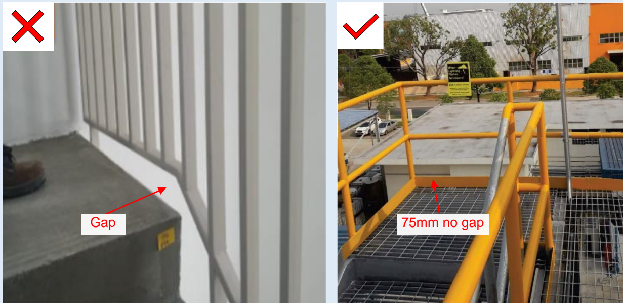
Figure H—XXV: No gap at 75mm from FFL is applicable to M&E areas
