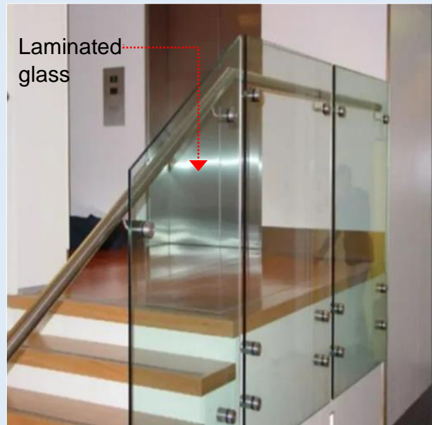
Figure H—III: Laminated glass (indoor) in a house built for owner’s own use
