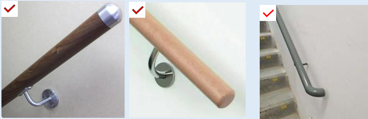
Figure E—XXII: Acceptable rounded off handrail that returns to the wall (Only for residential units including landed houses)
