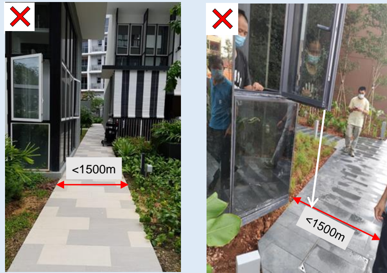
Figure C—XII: Openable windows found in public access space that reduced the required width of accessible route
