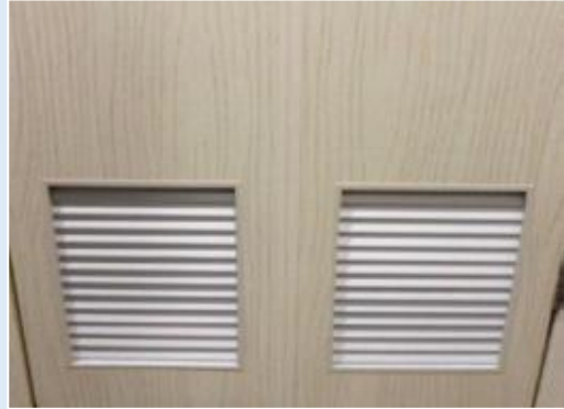
Figure G—X: Openings in fixed louvres
