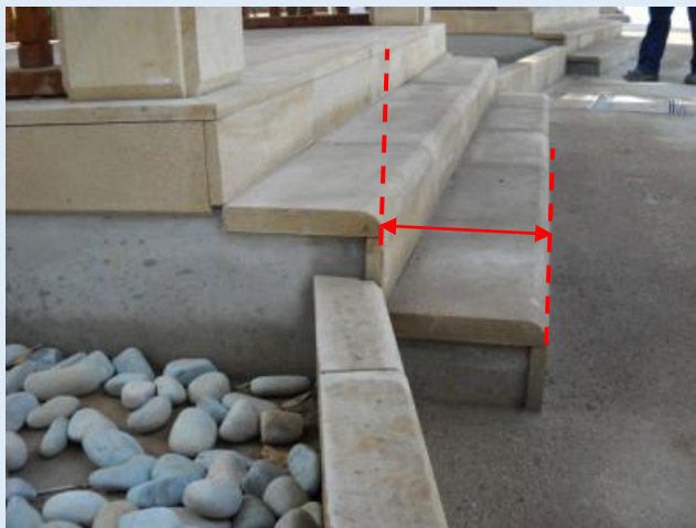
Figure E—II: Measurement of tread with rounded nosing
