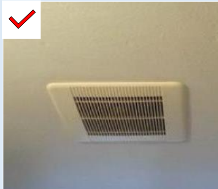
Figure G—IV: Ducted fresh air supply outlets
