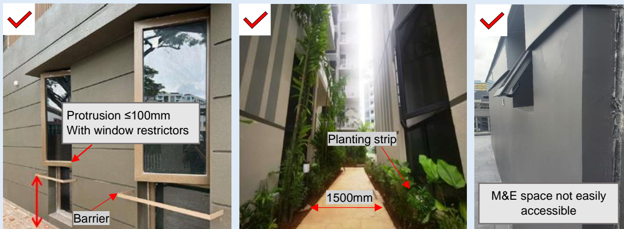
Figure C—XIII: Barriers and planting strips are some of the acceptable measures for public circulation space
