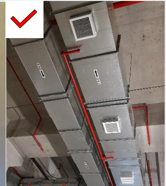
Figure G—IV: Ducted fresh air supply outlets
