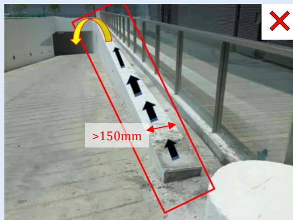
Figure H—XXII: Kerb along carpark ramp poses danger of falling from height
