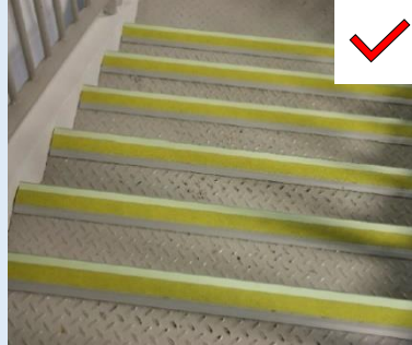
Figure E—XXV: Nosing provision for perforated metal staircases at maintenance areas
