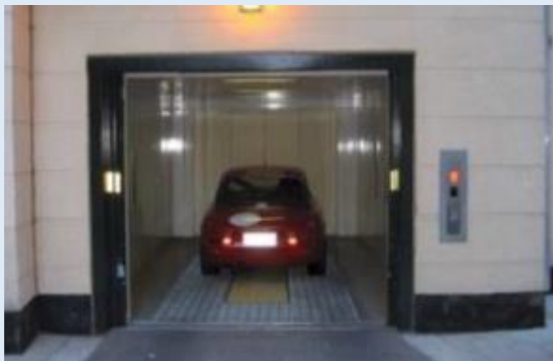
Figure K—I: Car lift intended to convey vehicles together with driver/ passengers
