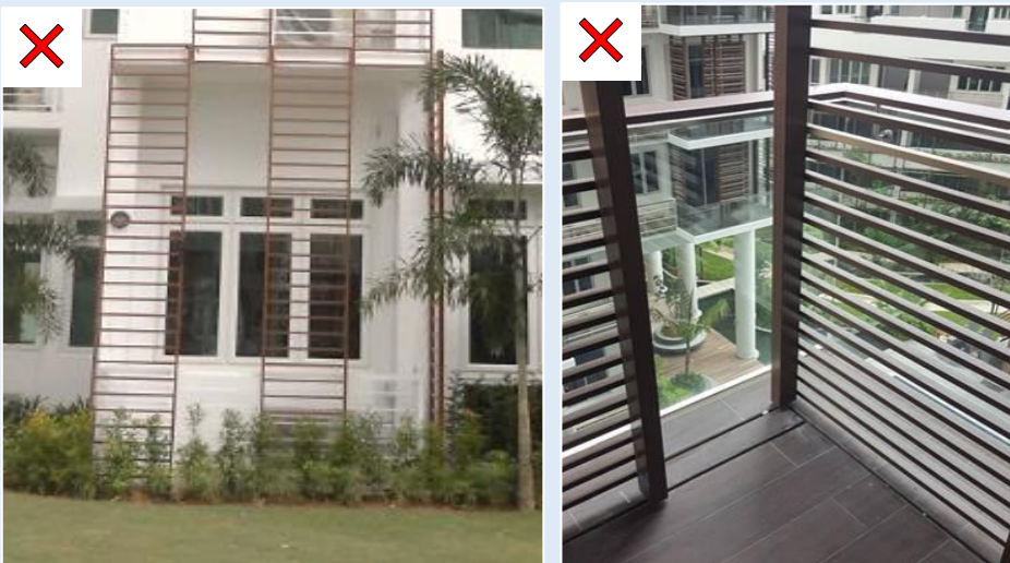
Figure H—1: Climbable features posing risk of falling from height
