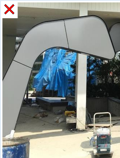
Figure C—VII: Slanted structure at gym area was straightened
