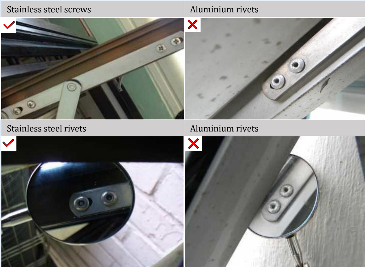
Figure M—1: Window fasteners
