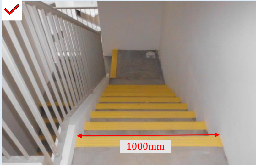
Figure E—VII: Measurement of the width of staircase with protruding kerb
