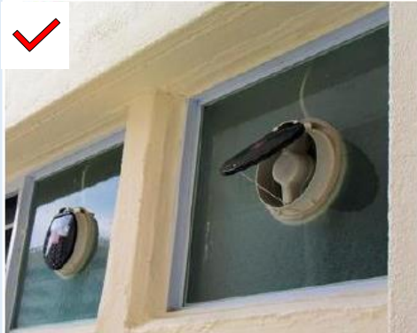
Figure G—III: Window or wall mounted fan
