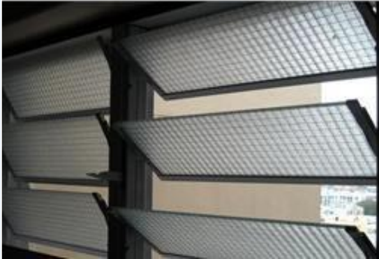
Figure G—IX: Openings in adjustable louvres
