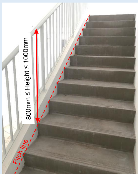
Figure E—XII: An example on the measurement of height of handrail from pitch line
