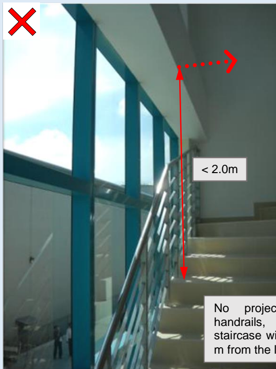
Figure C—XVII: Examples of headroom non-compliances along staircases
