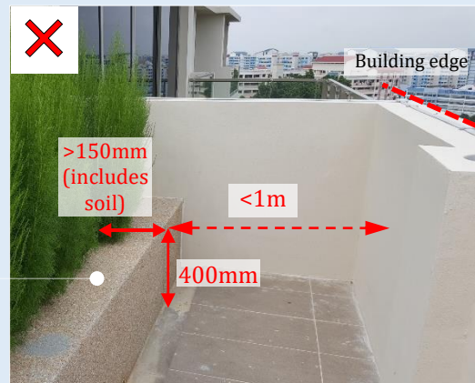
Figure H—XIX: Explanation of flat climbable surface less than 1000 mm away from the top of the barrier
