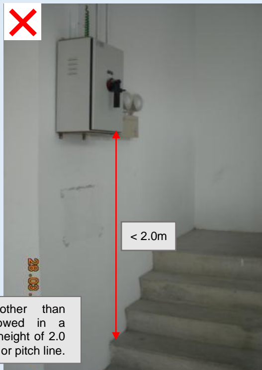
Figure C—XVII: Examples of headroom non-compliances along staircases
