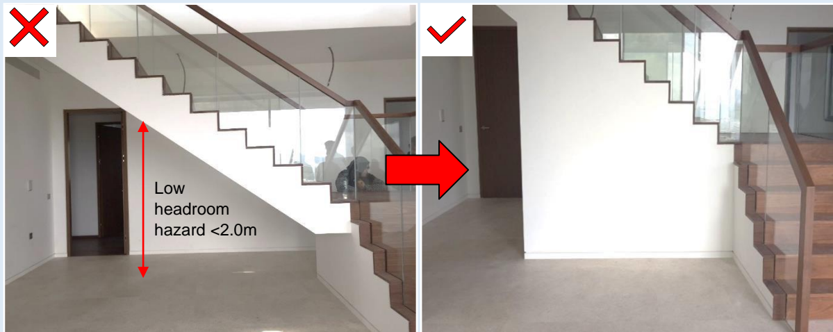
Figure C—II: Low headroom at entrance is mitigated by building up a storage area underneath the staircase
