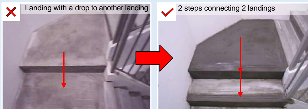
Figure E—X: An example of landing with a step being rectified
