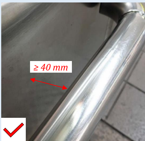
Figure E—XVII: Clear space from smooth wall surface (Min. 40mm wall gap)
