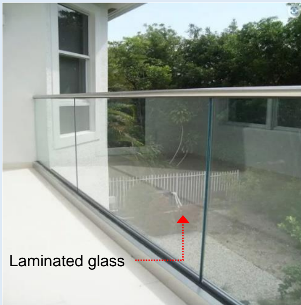
Figure H—II: Laminated glass (outdoor) in a house built for owner’s own use
