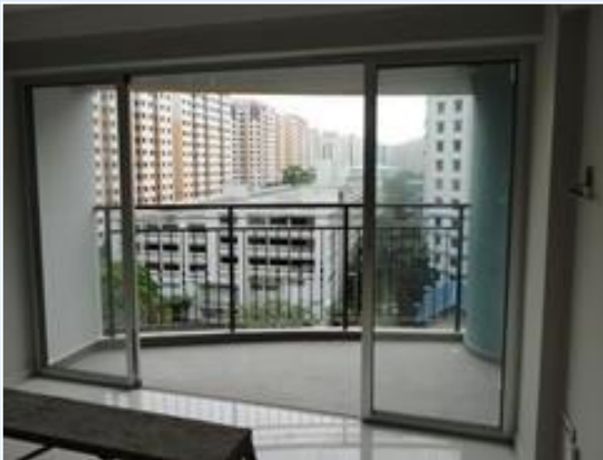
Figure G—XI: Openings in balcony
