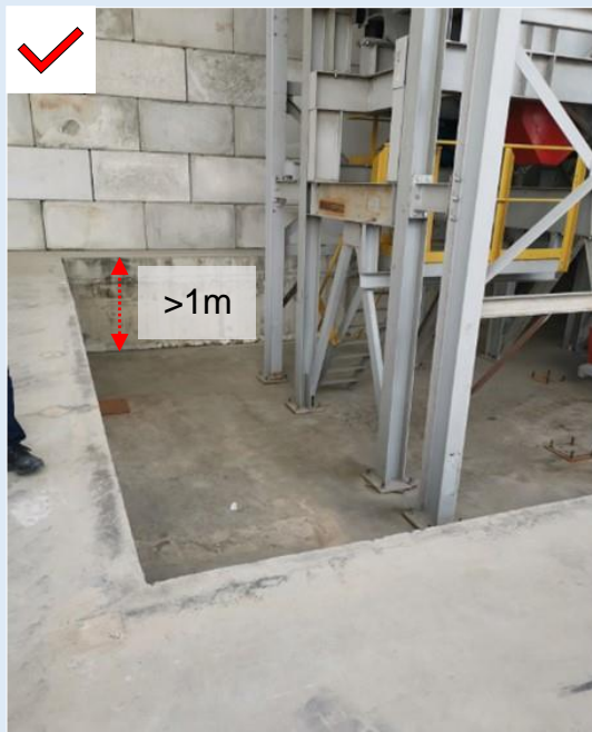
Figure H—XII: M&E floor openings without barriers
