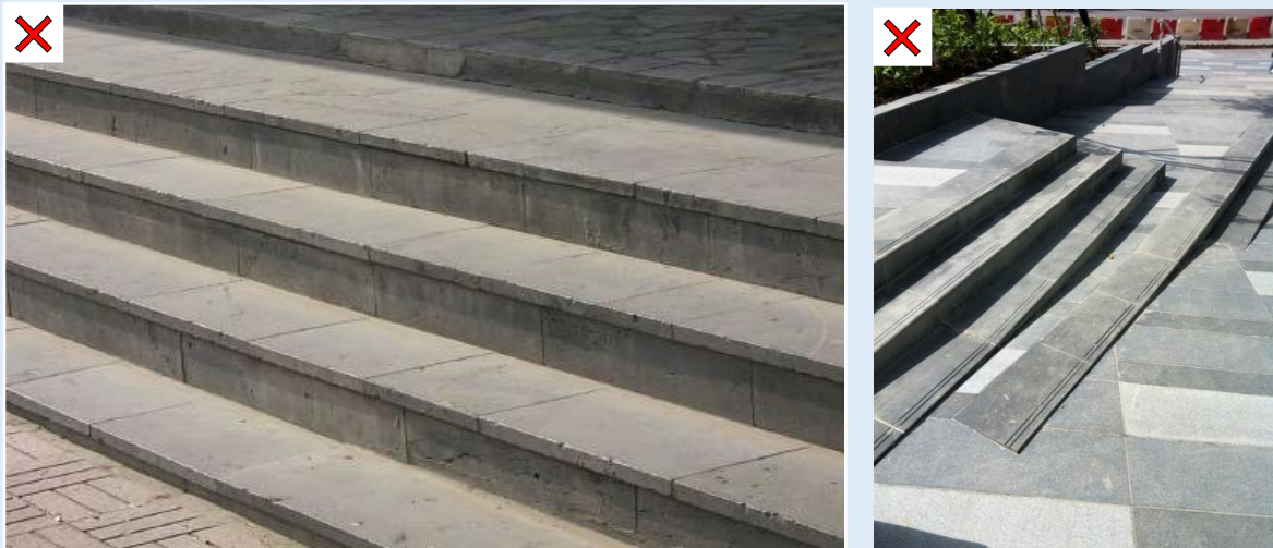
Figure E—V: Examples of irregular risers
