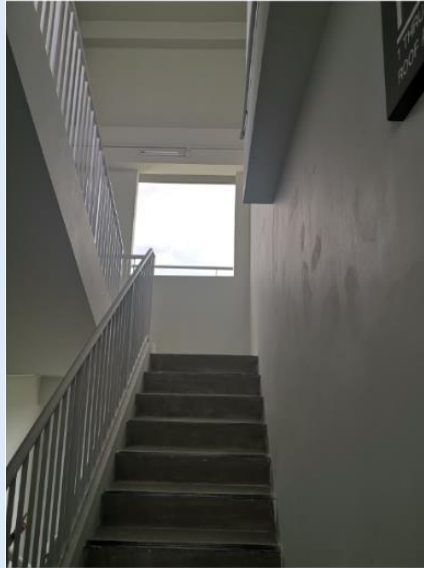
Figure H—V: Staircase to the Roof
