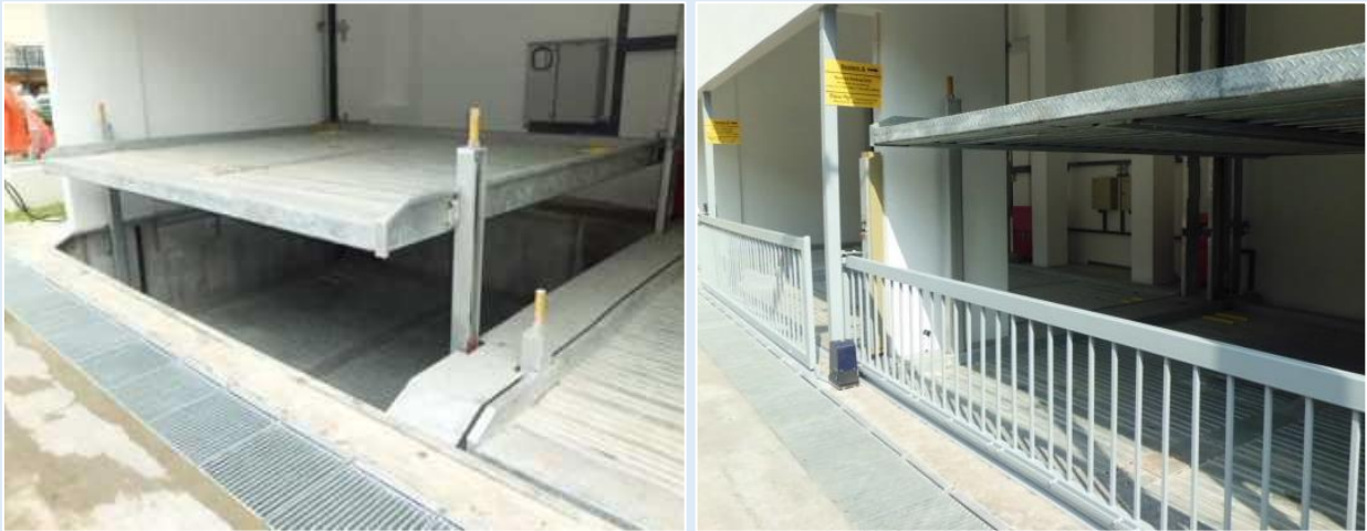
Figure A2—III: The risk of fall at the MCPS is being mitigated with barriers
