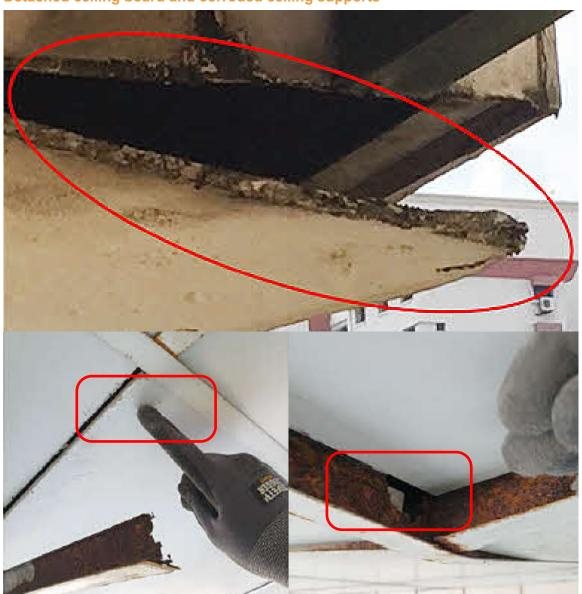
Detached ceiling board and corroded ceiling supports
