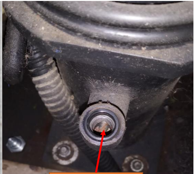
Insufficient Hydraulic Oil
