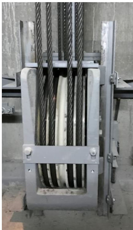
Compensation rope sheave tie-down
