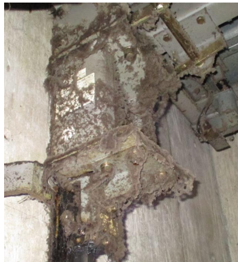
Poor housekeeping of lift pit and hoistway
