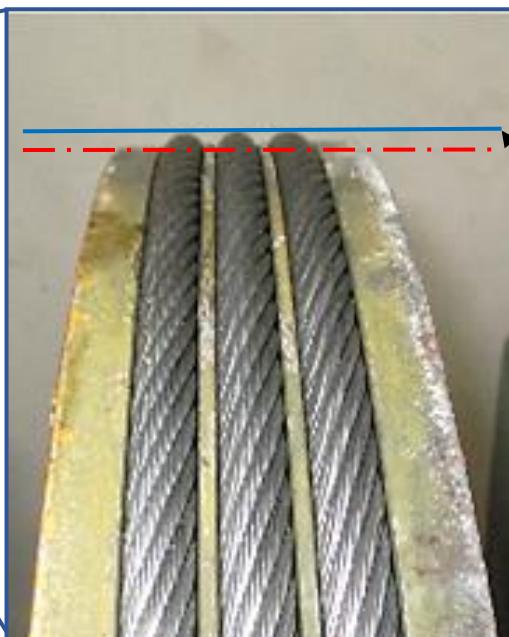
Rope on sheave
