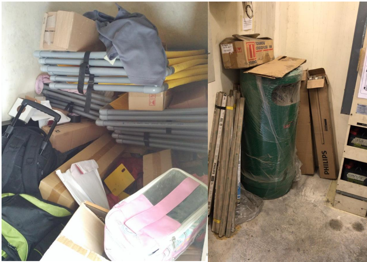
Poor housekeeping of motor room
