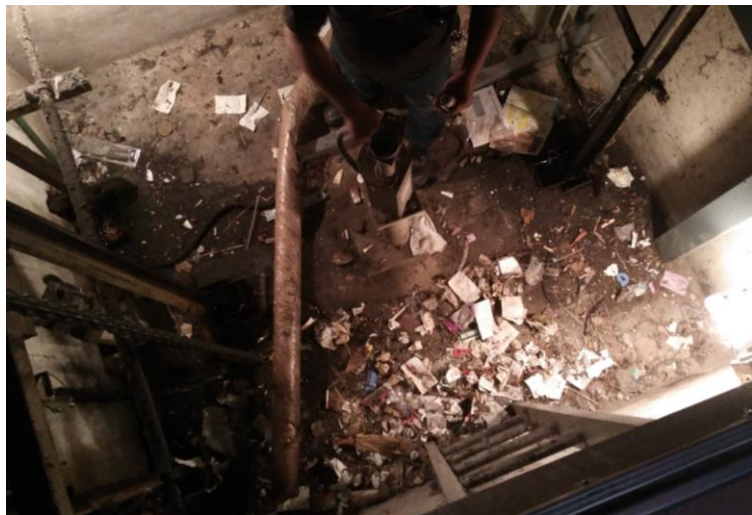
Poor housekeeping of lift pit and hoistway
