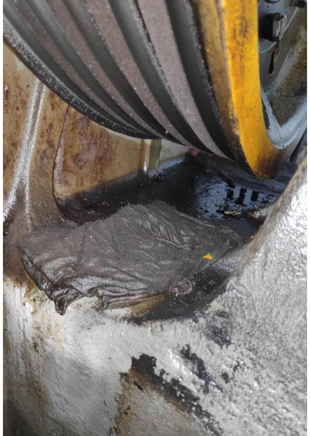
Oil leakage at lift machine and drive
