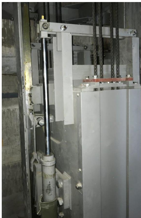
Compensation rope sheave tie-down
