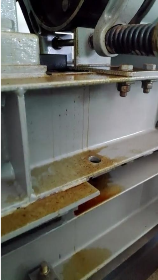
Oil leakage at lift machine and drive
