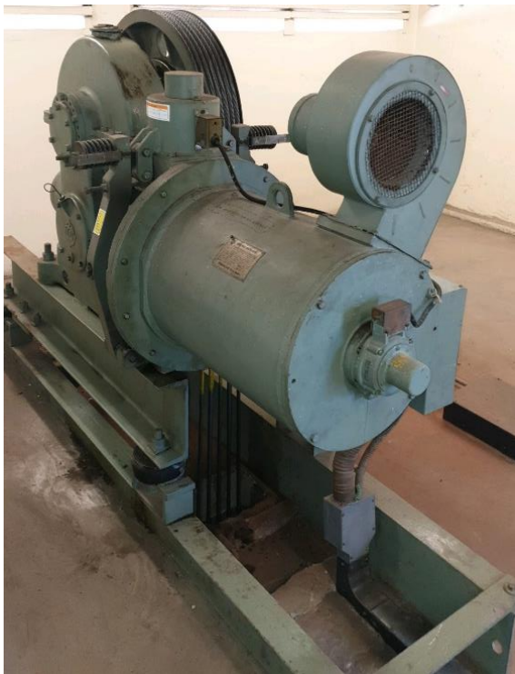
Secure lift machine and drive
