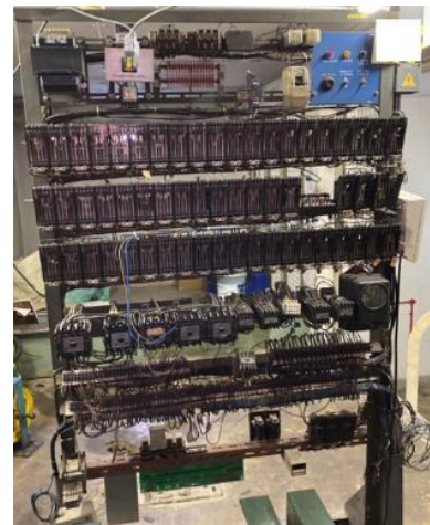
Figure 3: Outdated Lift Controller
