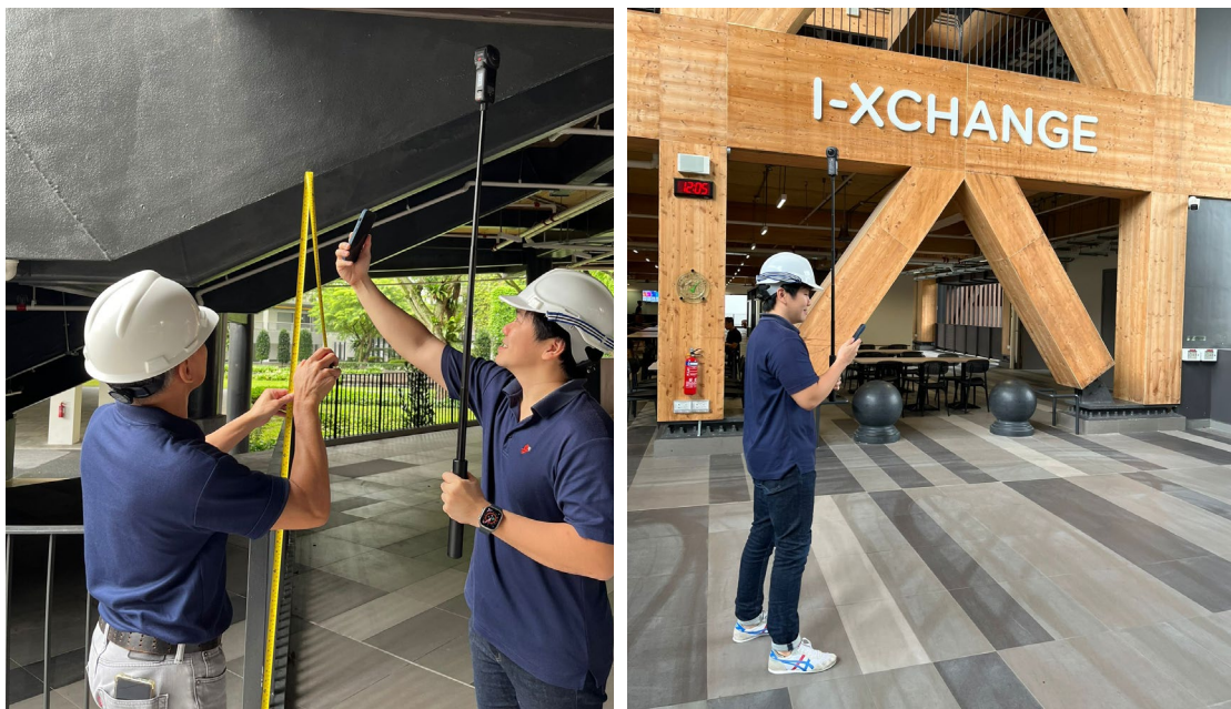
Pictures 1 and 2: Virtual inspections can be done using 360 capture devices to record site findings.
