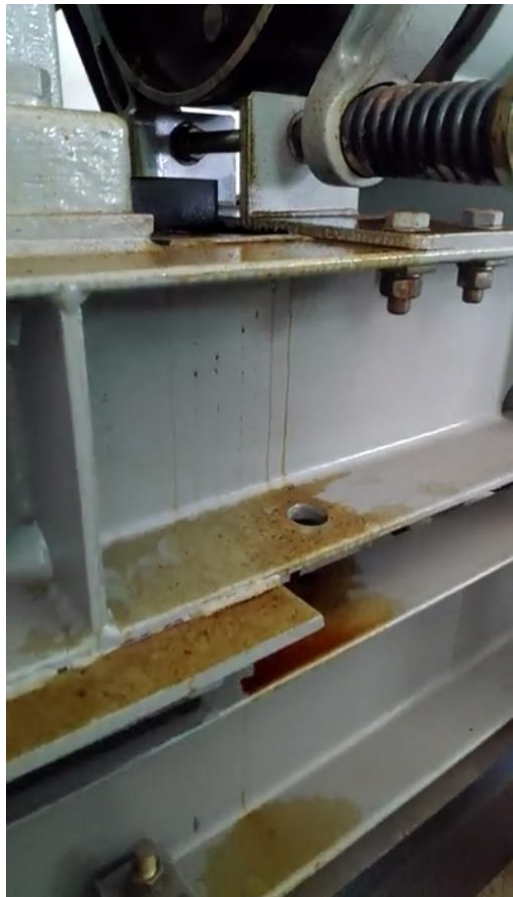
Oil leakage at lift machine and drive
