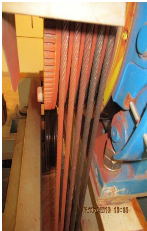
Rust on lift machine
