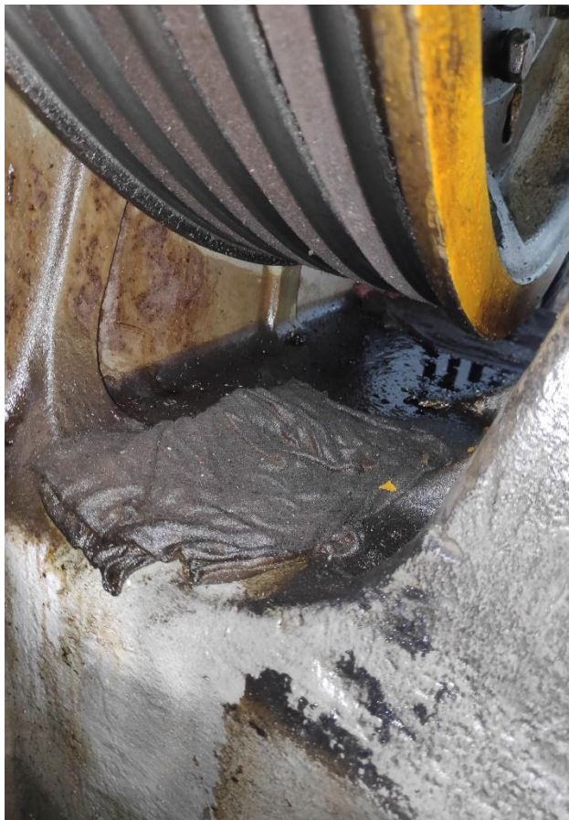
Oil leakage at lift machine and drive
