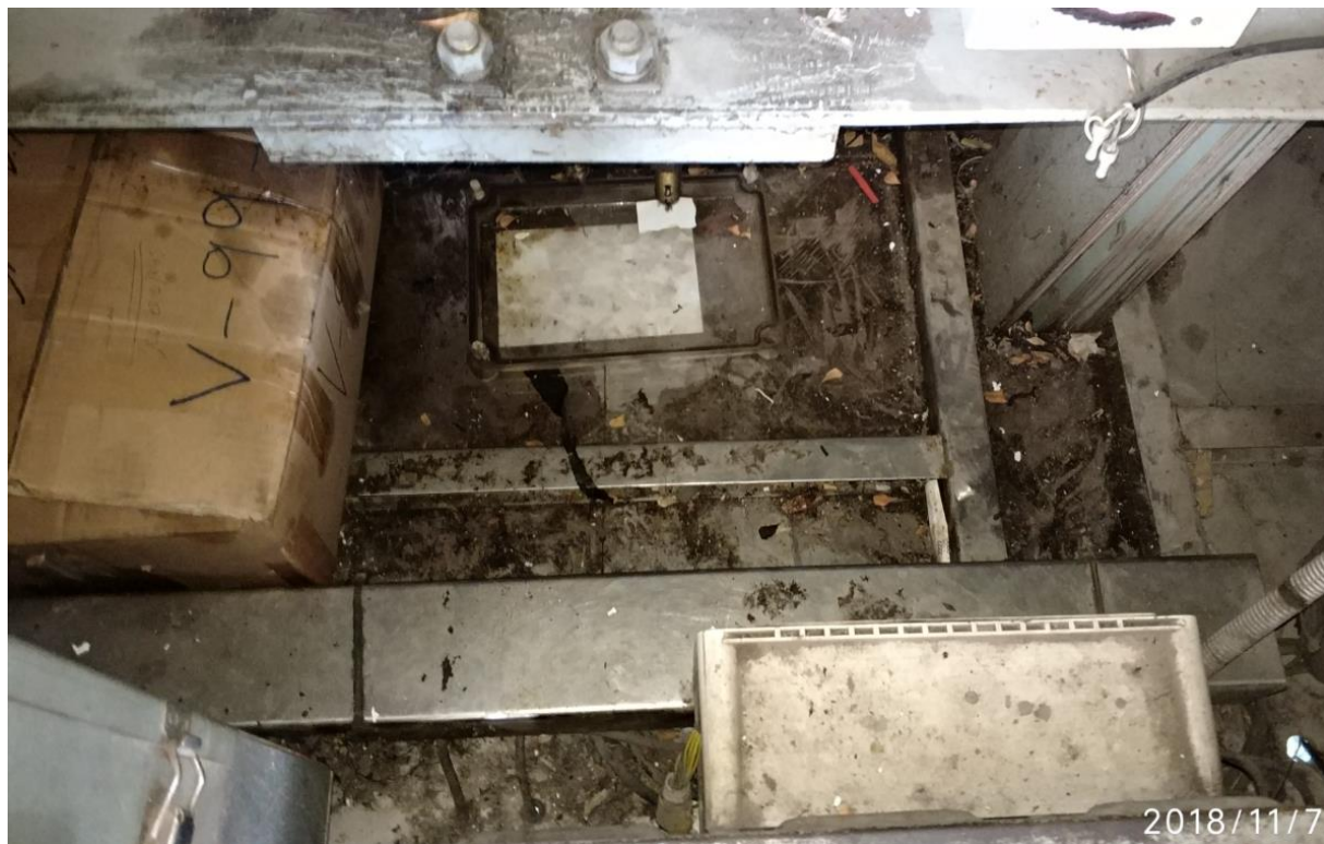
Poor housekeeping of lift car top
