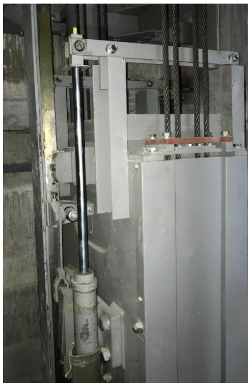
Compensation rope sheave tie-down
