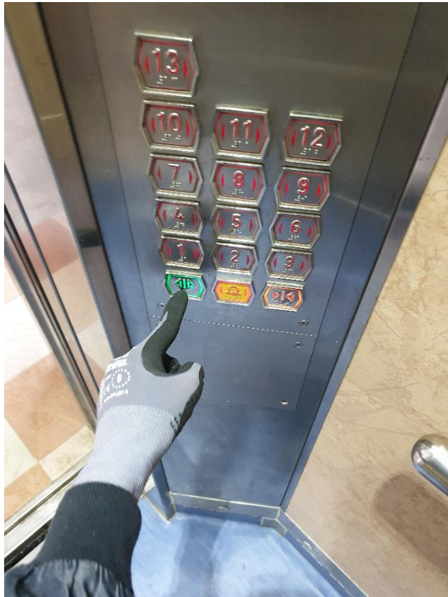
Door open button check - lift car
