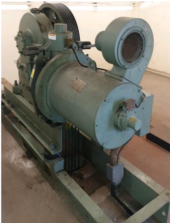
Securely mounted lift machine and drive
