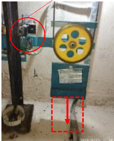
Governor rope tensioning sheave
