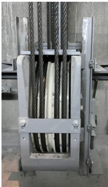
Compensation rope sheave tie-down
