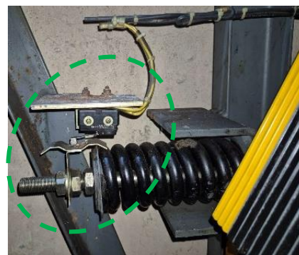
Step chain tensioning switch
