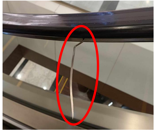
Sharp Protrusion
