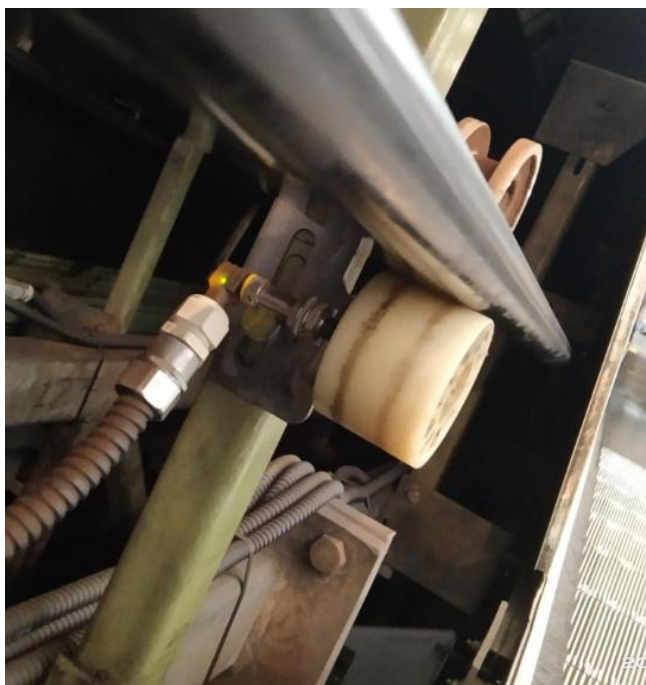
Handrail speed monitoring device
