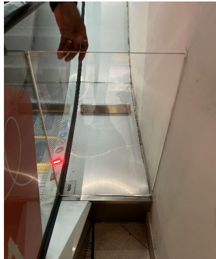
Loose anti-climb panel
