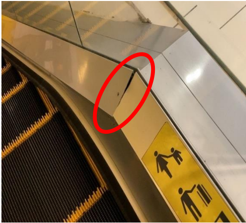
Sharp edges on skirt panel
