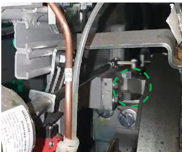
Auxiliary Brake Position 1 - Lock Position
