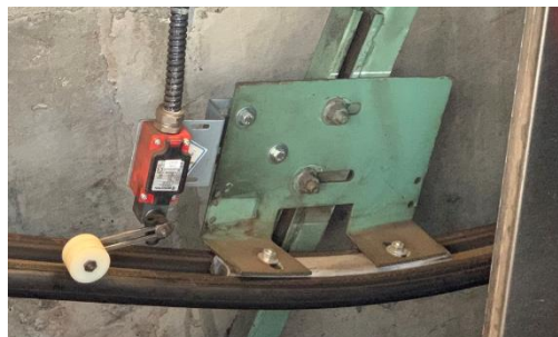
Handrail breakage switch
