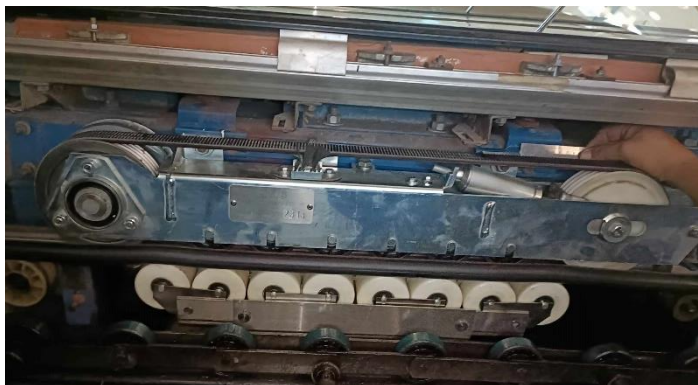
Handrail drive belt properly tension and maintained
