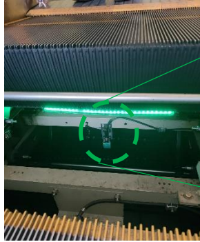
Missing step detection device
