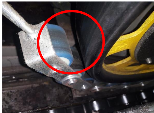
Rollers not in contact with the handrail belt
