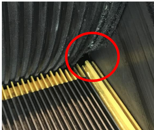
Damaged step (riser)
