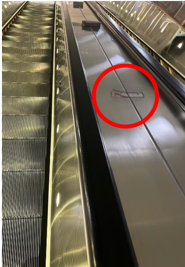
Missing anti-sliding bump
