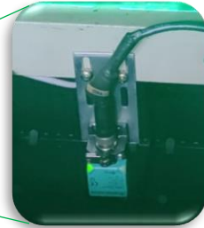
Missing step detection device
