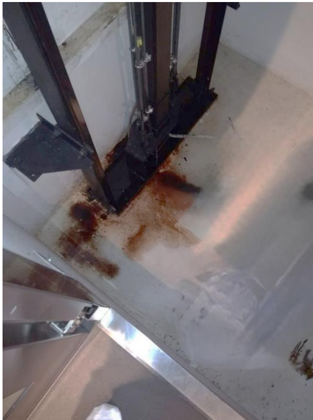
Oil accumulation in lift pit
