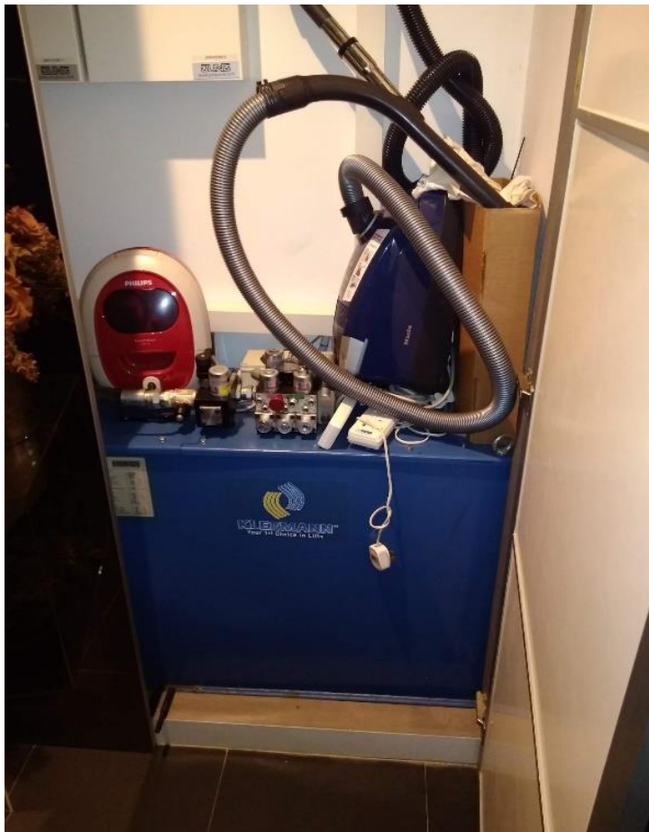
Poor housekeeping of machinery space
