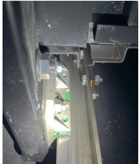
Guide holder and guide shoe are intact
