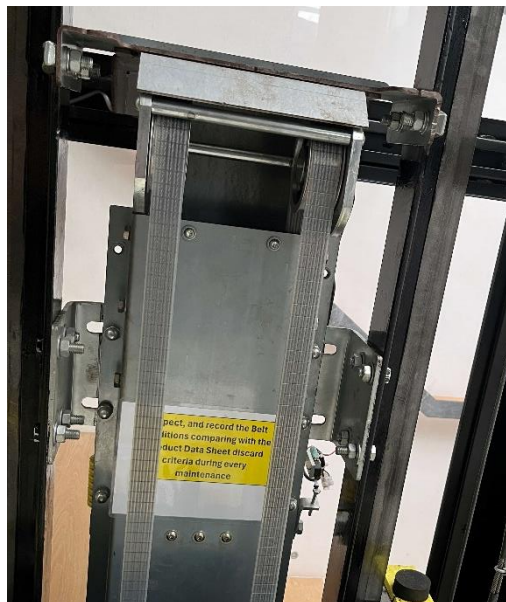
Belt drives are equally tensioned
