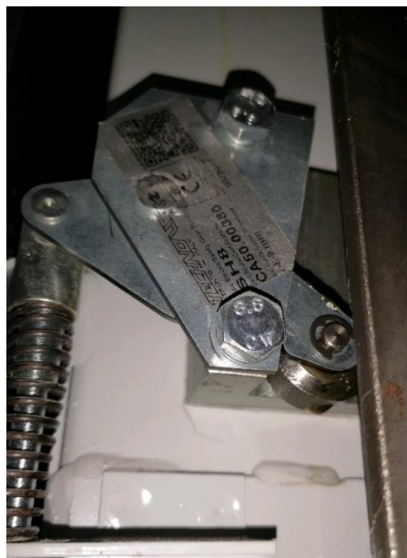
Safety gear components
