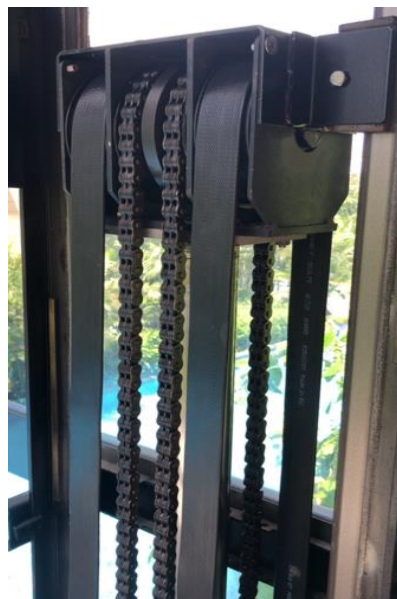
Chains are not broken or elongated
