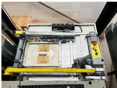
Mechanical blocking device at lift car top
