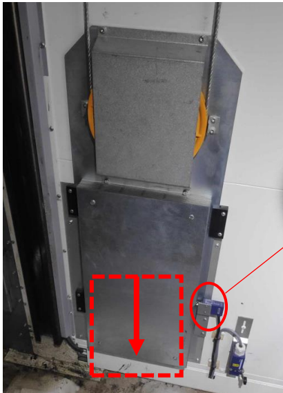
Governor rope tensioning sheave
