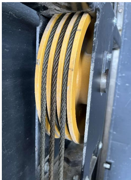
Main ropes are properly tensioned
