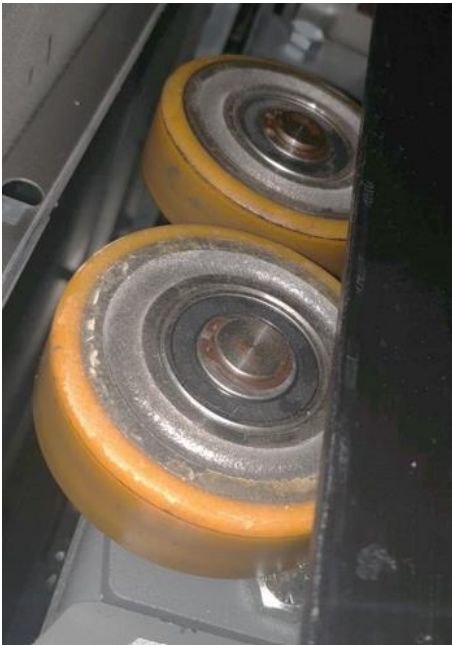
Roller guides lining is intact
