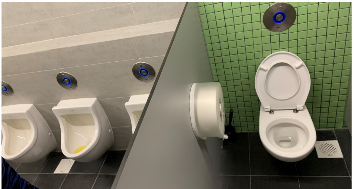
Photo (above): Example of child-sized urinals and water closets to promote independent usage.
