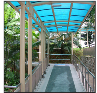
Landings provided at the change in direction
