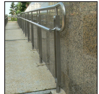
Handrails of two varying heights with extension at the end
