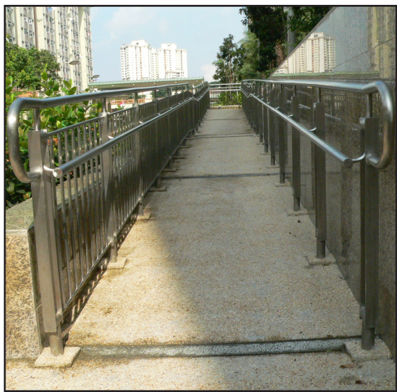
Ramps for universal access should be of consistent and gentle gradient, with adequate landings.
