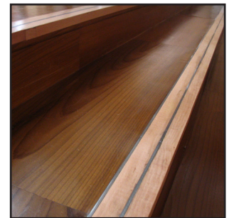
Special non slip nosing of permanent contrasting colour
