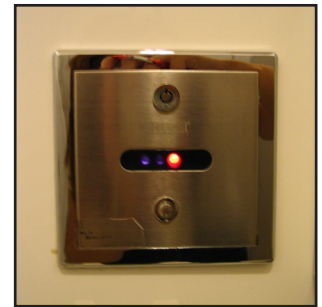
Automatic flush sensor
