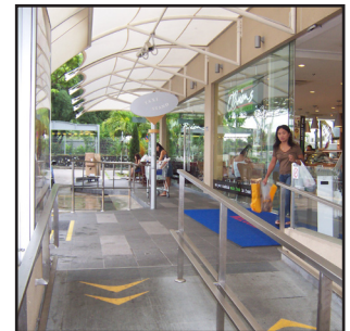
Minimum clear width of 1200 mm
