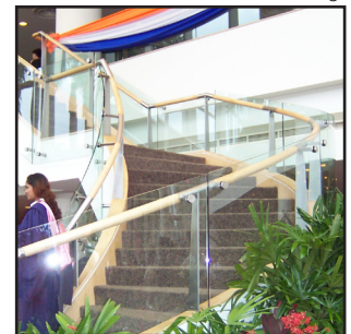
Circular stair with an acceptable minimum tread dimension
