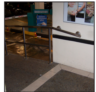
Handrails extension at the end of the run
