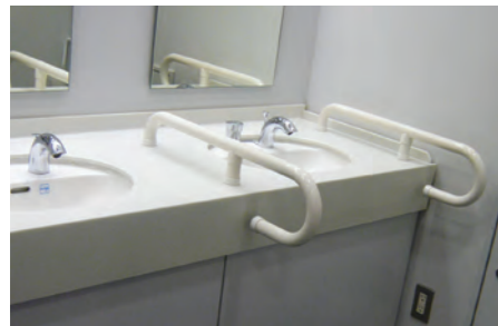
Photos (above): Well-designed toilet with adequate illumination, non-slip floor finishes and well-placed toilet accessories; wash basin with grab bars
