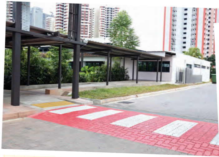
➔ Strong colour contrast with the surroundings for greater visual clarity (applied where there is change in levels, as well as between walls, floors, furniture or fittings)
