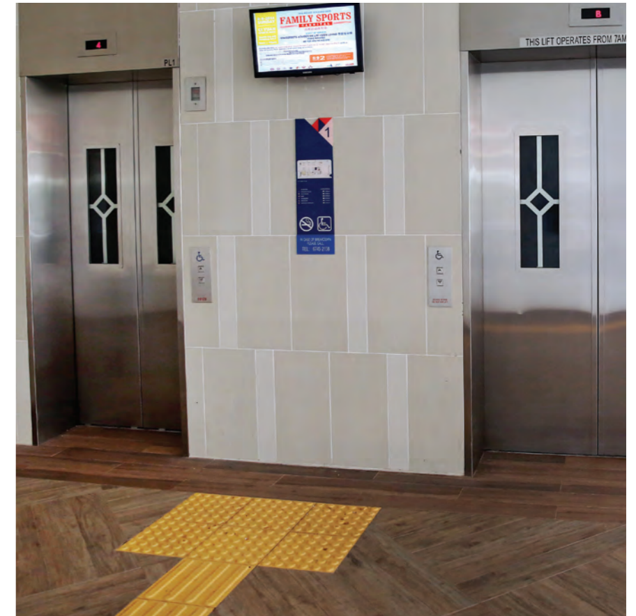
Photo: Lift lobby with tactile ground surface indicators leading to accessible lifts with vision panels
