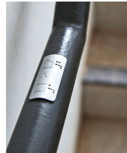
Photo: Braille and tactile information on handrail
