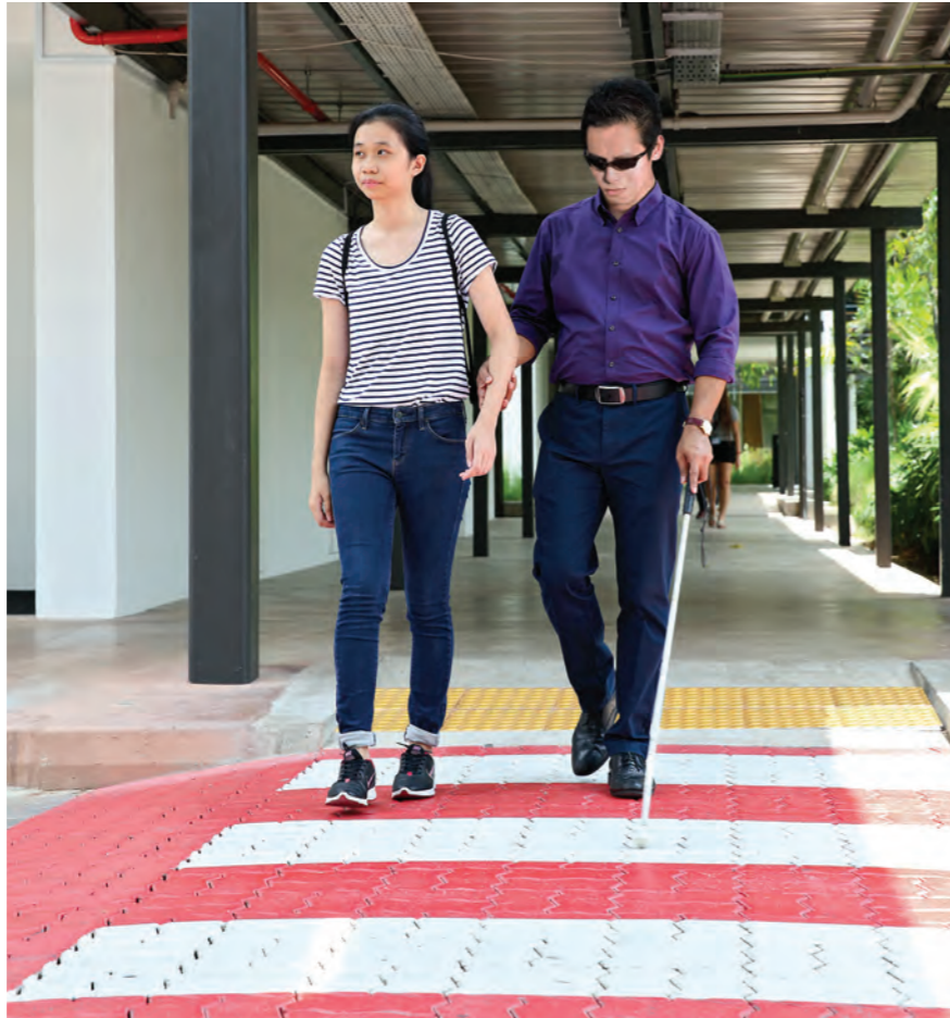
Photo: Detectable warning surfaces at a pedestrian crossing
