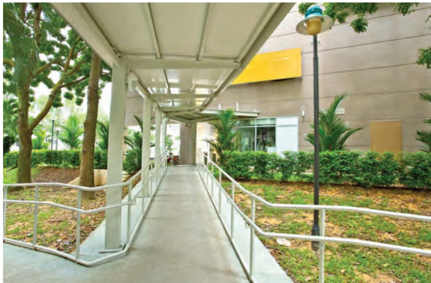
Photos (right): Examples of accessible entry to the community club
