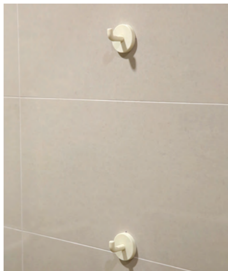
Photos (above): Designated hooks for walking sticks and bags near wash basins; recessed hand dryers and waste bins; a pair of coat hooks in WC compartment
