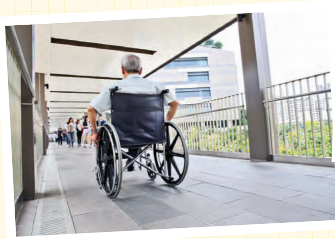
➔ Ramp with a gentler gradient and non-slip floor surface
