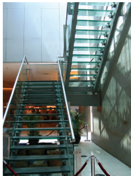
Photo: Open risers and transparent treads that should be avoided
