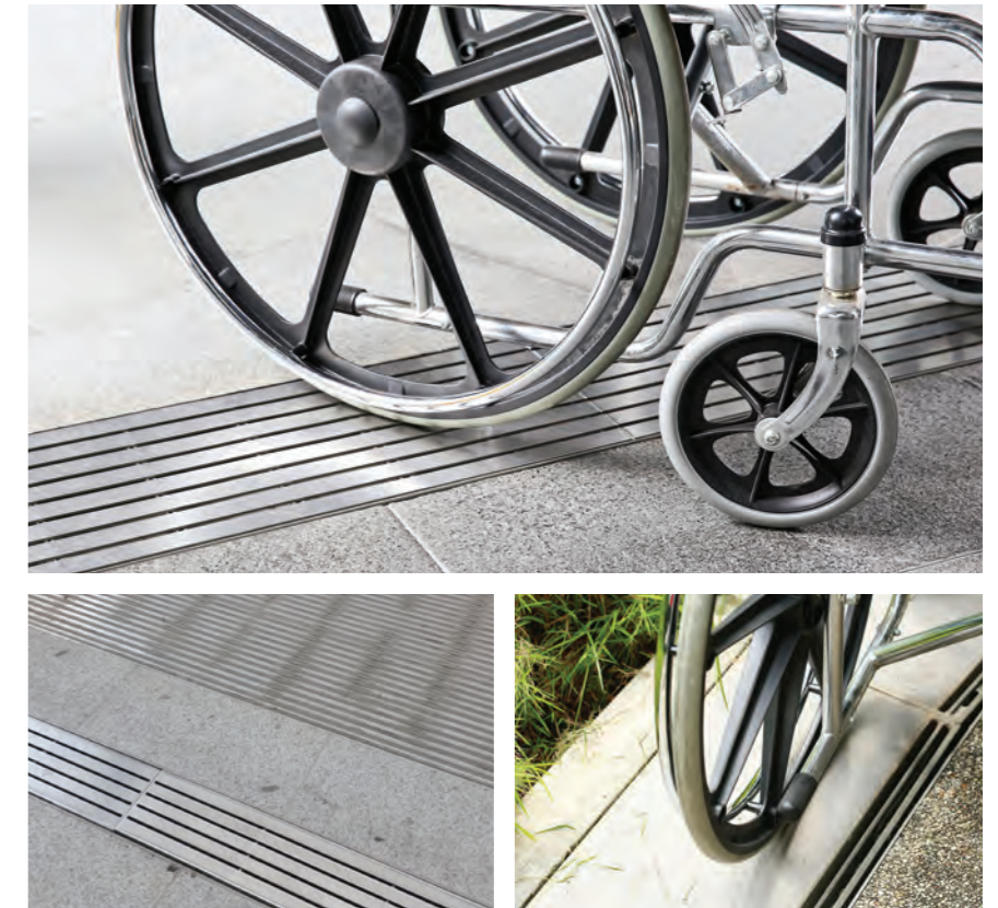
Photos (right): Examples of gratings and drain covers with appropriate slots and gaps
