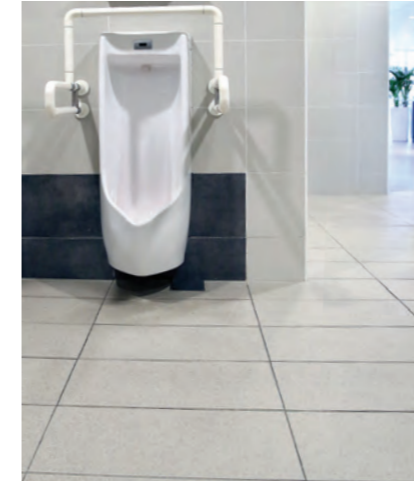
Photo: No steps or drop in level at toilet entrance and within toilet area
