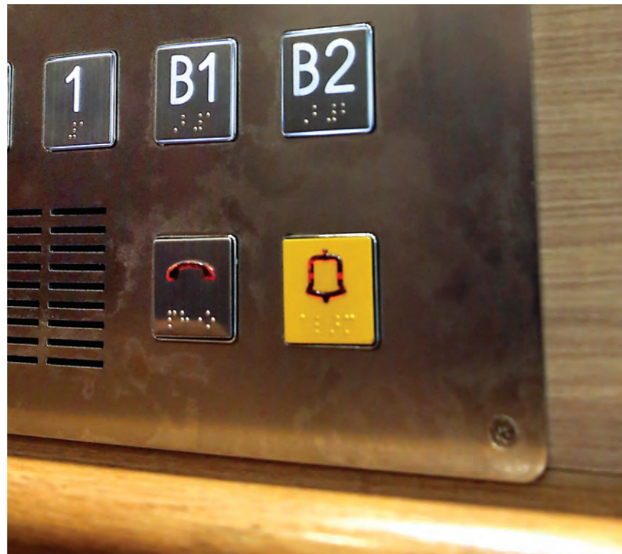
Photos (above): Tactile ground surface indicators on the floor surface at a lift lobby; an emergency bell button
