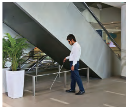
Photo: Detectable guardrail under escalators
